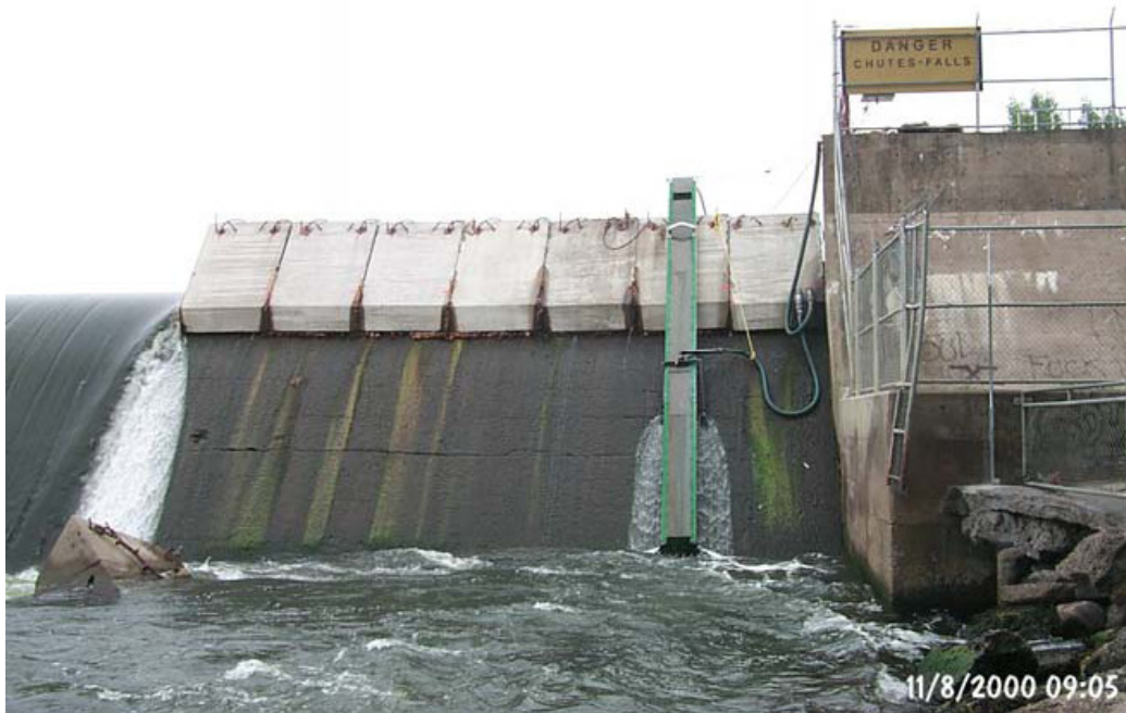
Figure 4 Photograph of the ladder
