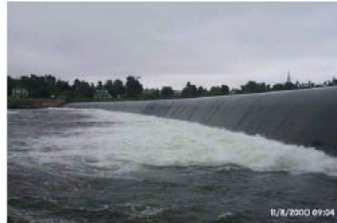
Chambly Dam on the Richelieu River
