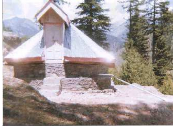
Fig.-6 Water Supply Plant
