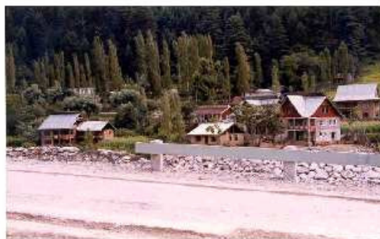
Fig.-4 Reconstructed Houses
