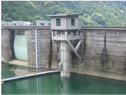
Photo 1 Intake tower of outlet structure for compensation flow
