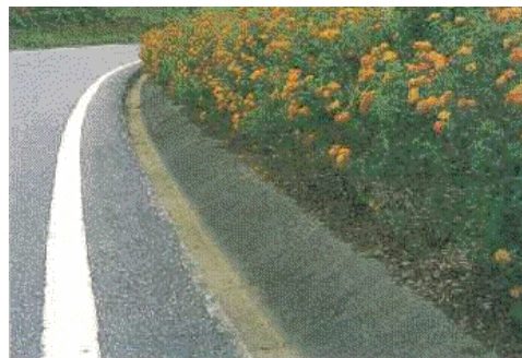
Fig. 5 Slope-type side ditch
