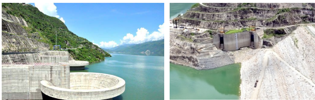
Figure 48 Spillways: Clockwise from top Chute (1 & 2), Left Bank Shaft & Right Bank Shaft Spillways
