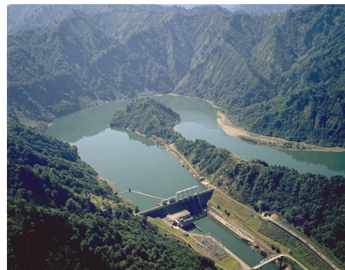
Entire View of the Taki Power Plant and the Taki Dam
