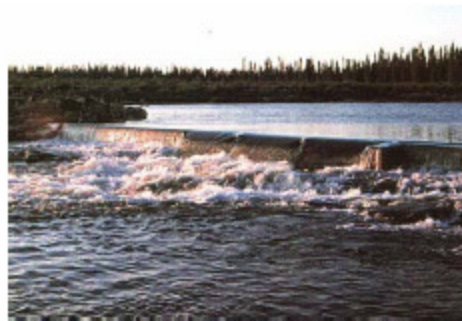
Fig. 17: Concrete weir with control structure Vincelotte River
