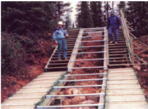
Fig. 9: Portage with hauling structure Vincelotte River
