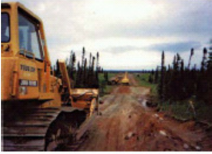
Fig. 7: Construction of the Vincelotte access road
