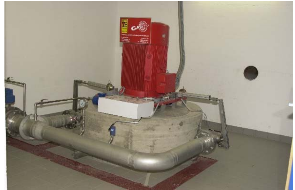
2-nozzle Pelton turbine H_n = 105 \text{ m} , Q = 90 \text{ l/s} 580'000 kWh/year - Production sold to the grid
