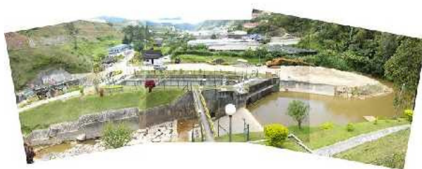
Photo 1 Desander in front of the Telom Intake
