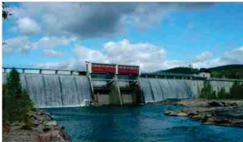
The intake pond Eikredammen has limited storage capacity (0.4 Mm 3 )
