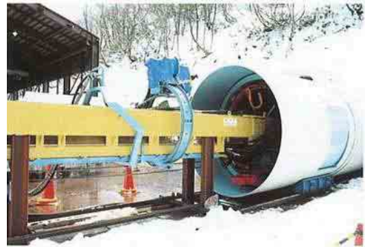
Fig. 6: Shotcrete Robot behind TBM
