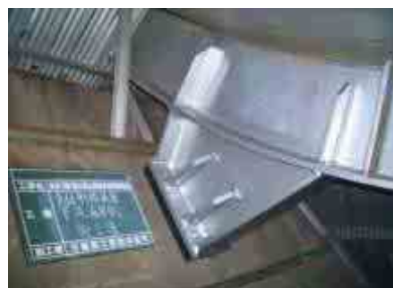
Fig. 7: Outline of Aseismic bearing construction of the Water-tube bridge
