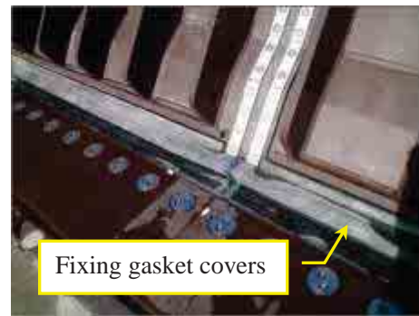
Photo 6: Rubber gasket covers
