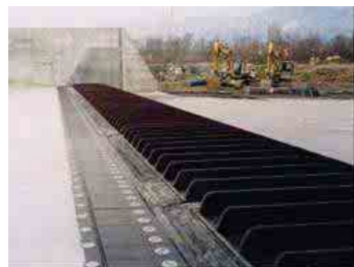
Photo 5: SR dam lying completely flat
