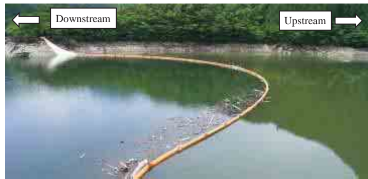
Photo 1: Installation status of the Fence as a countermeasure to muddy water
