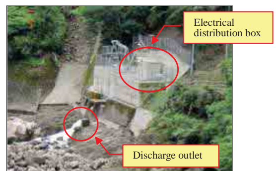
Fig. 8: Installing status of the distribution box
