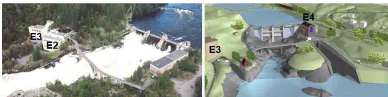
Arrangement of old (E2 and E3) and new (E3 and E4) power houses
