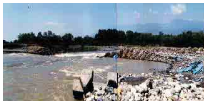
Photo 4: Wash out loss of the dam after flood
