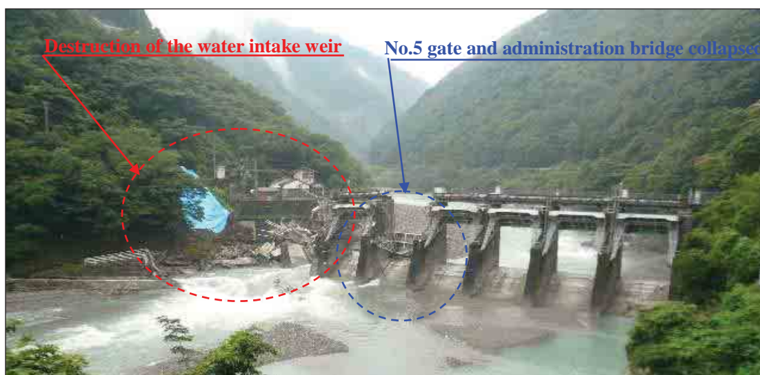
Photo 2: Distant view of the destruction of the water intake weir
