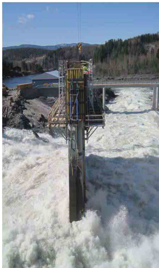
Construction of center dam pillar during flood, 2011
