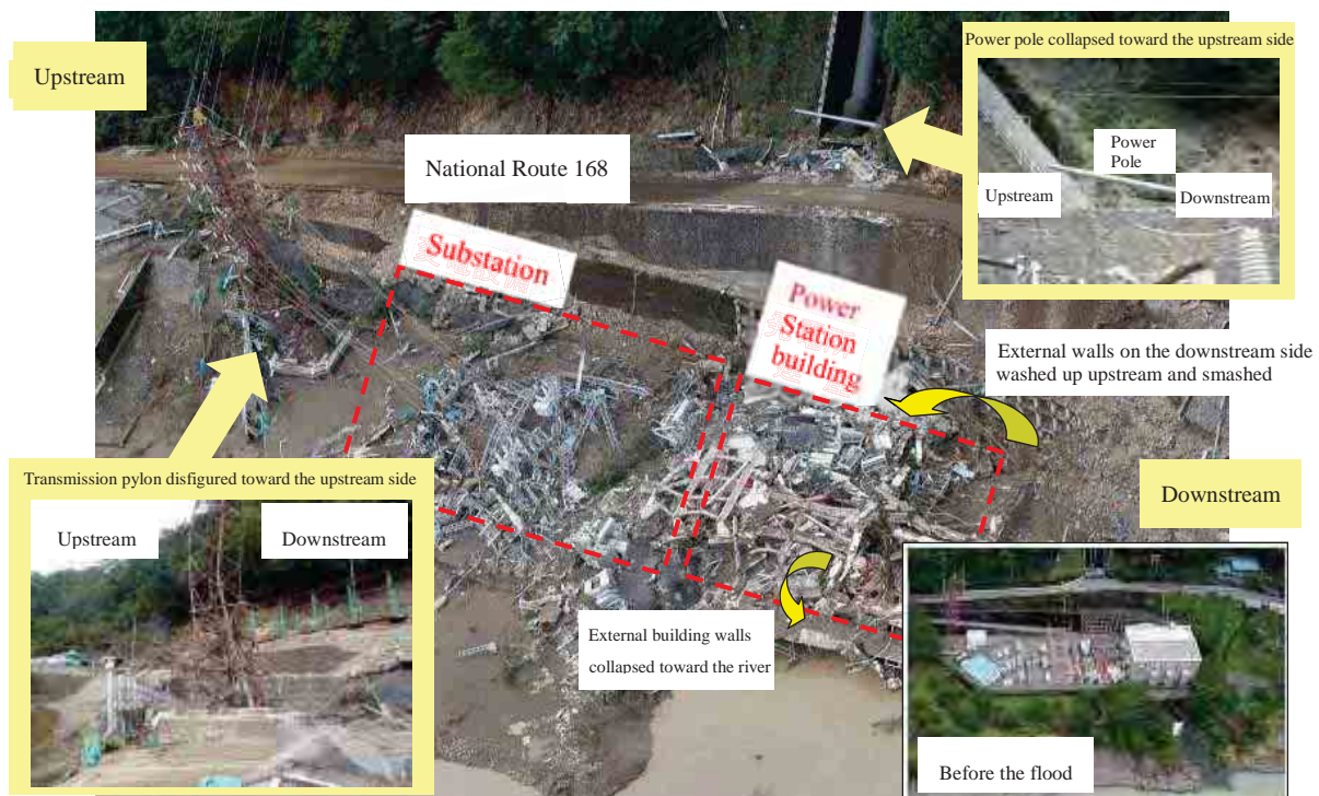
Fig. 2: Damage status of the Nagatono Power Station
