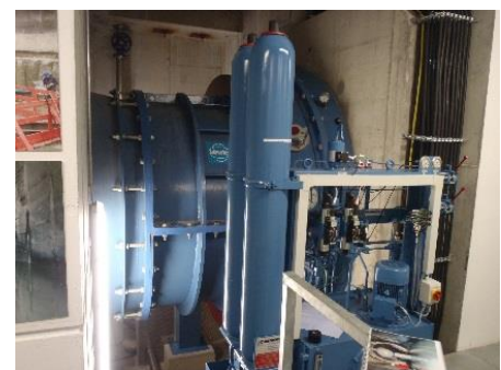
Photo- 2 Internal view of power plant (Turbine in back; hydraulic unit in front)
