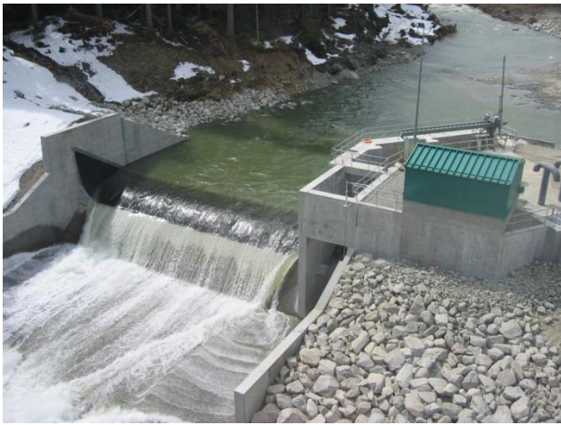
Photo-1 Diversion Weir and Intake [2]
