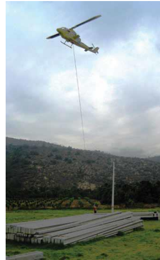
Photo-4 MW line erected by helicopter [2]
