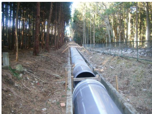
Pipeline (under underground installation)
