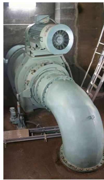
Photo-8: Water turbine and generator (after the renovation)
