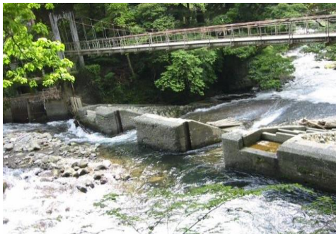
Photo-1: Intake weir and intake (before the renovation)
