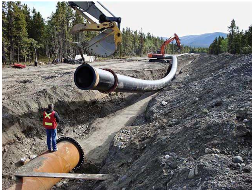
Photo-2. HDPE Penstock during construction [5]
