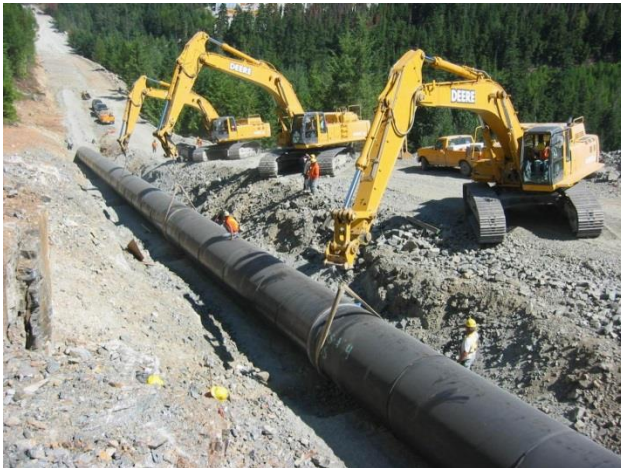
Photo-3. Buried Steel Penstock Construction [2]
