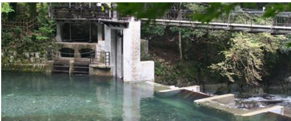
Photo-2: Intake weir and intake (after the renovation)
