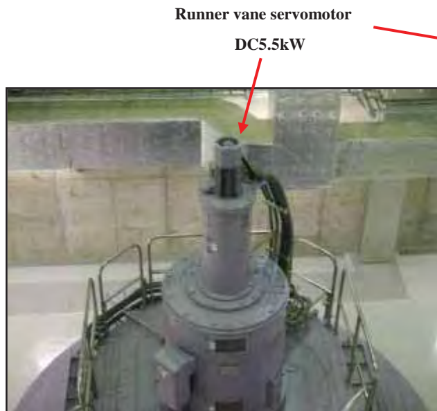
Photo 4 Runner vane servomotor
