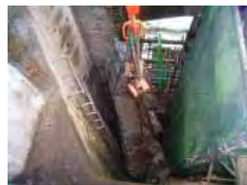
Photo. 4 Hoisting of the blocks
