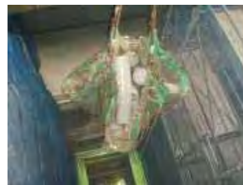
Photo. 2 Hoisting of the cut hole cores
