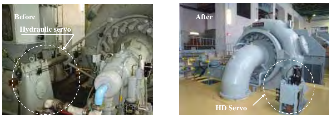
Fig.2 Pressure oil servo before the renewal and HD servo after the renewal
