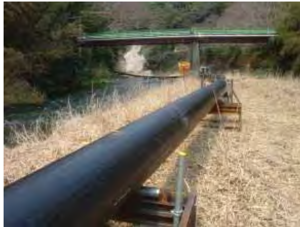
Photo 5 View of the pipe pulling in the works
