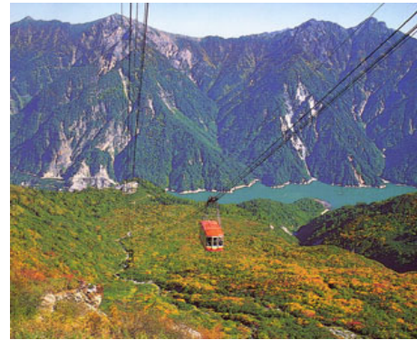
Fig.-5 The Rope way with Kurobe dam behind
