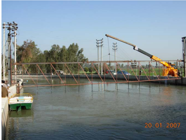
Fig. 17 (a) : Frame lowered to submerge PCMs into water
