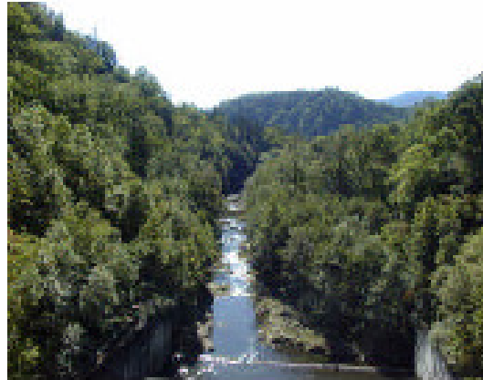
Fig.-6 Flow regime downstream of the Tomura Dam (September 2002)
