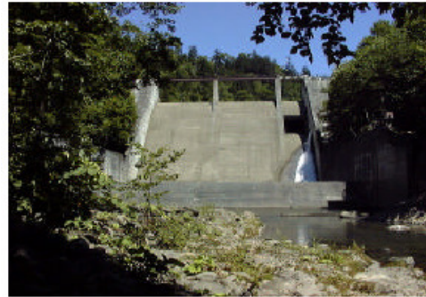
Front view of the Tomura Dam
