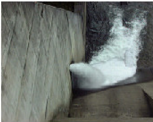
Fig.-5 The flow rate required to maintain the river functions (Tomura Dam)
