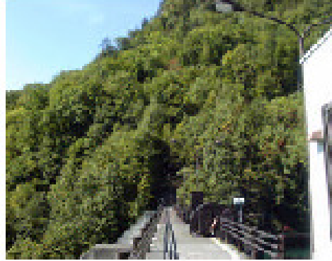
Fig.-11 Tomura Dam right bank area greened after completion of the project (September 2002)
