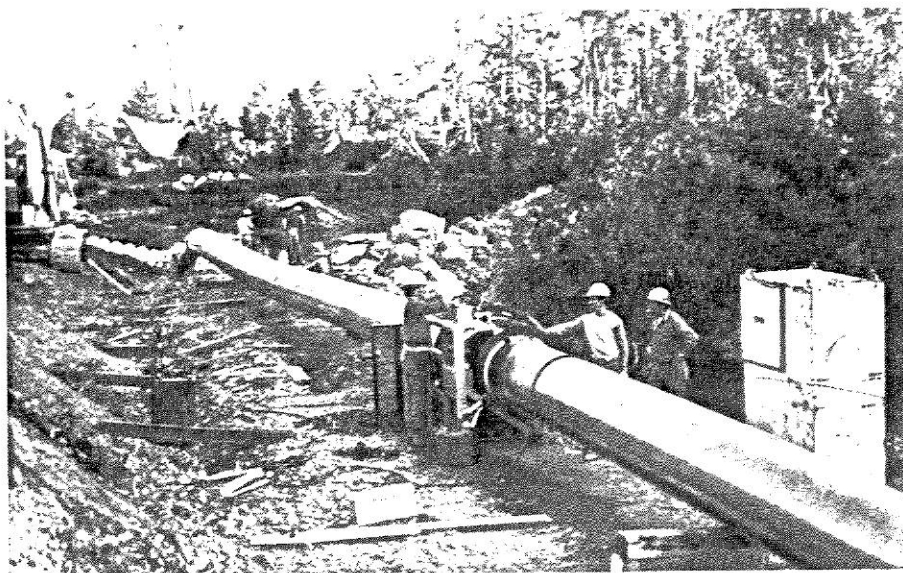
FIGURE 8: In New Richmond, Quebec, 28-inch internal diameter PVC pipeline was fuse-welded on-site. Five 50-foot long pipe sections were fuse-welded at the storage area before being towed into place along a prepared trench. Each 250-foot pipe section was then fuse-welded to the preceding pipeline section. Flexible pipeline was used at a stream crossing (top left of photo).
