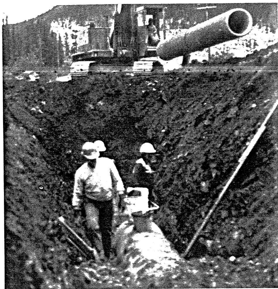
FIGURE 9: Buried concrete pipe located in Goat Creek, Alberta. This 2,200-foot long, 24-inch diameter pipe forms part of a pumping plant where local ground-water is pumped into the Spray power canal.
