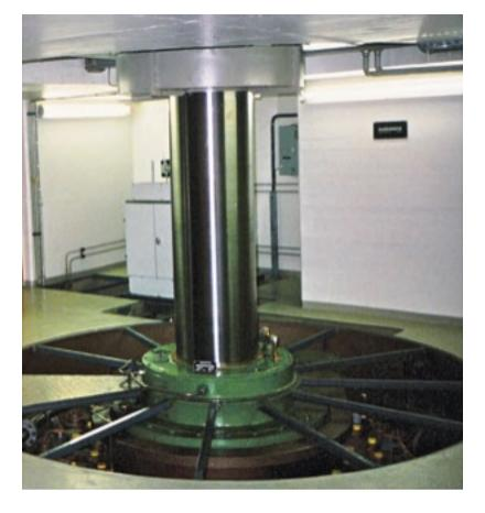
A common challenge at many hydro plants – no matter the size or location – is water leaking from the seal around the turbine's shaft. One solution to this challenge is using a seal with a face made of elastic polymer instead of carbon.
