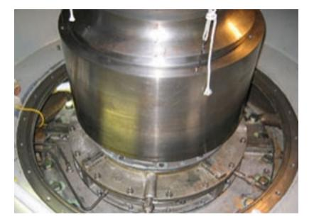
The new axial seal installed on this pump, at a facility in California, contains an innovative combination of face materials that can withstand severe applications. The old seal had to be replaced every three months; the new one has been in operation for three years.
