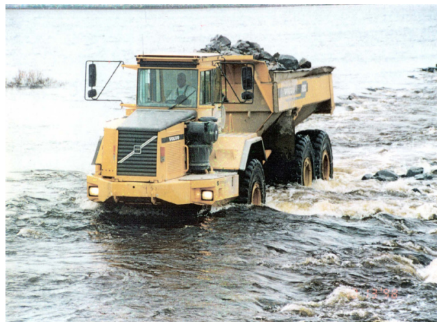
Figure 2 Weir under construction
