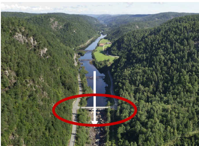
Across the river - impacting longitudinal connectivity
