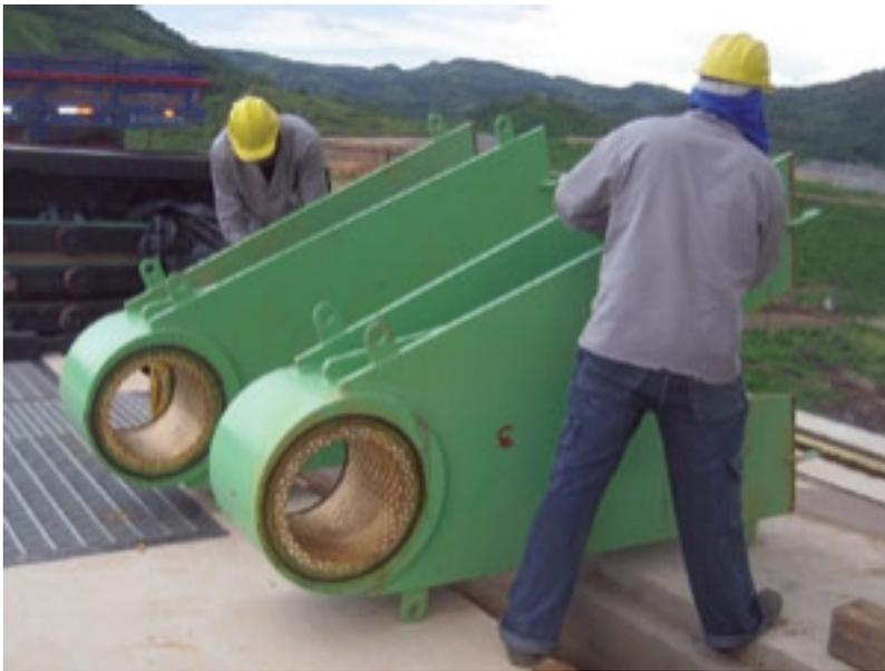
On these gate arms, the hydro project owner is using self-lubricated spherical bearings embedded with a polytetrafluoroethylene lubricant. These bearings are resistant to corrosion and do not present concerns regarding oil leakage into the water.
