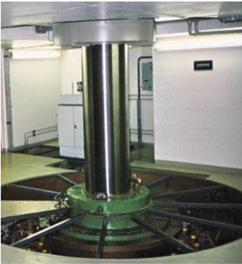
A common challenge at many hydro plants – no matter the size or location – is water leaking from the seal around the turbine's shaft. One solution to this challenge is using a seal with a face made of elastic polymer instead of carbon.
