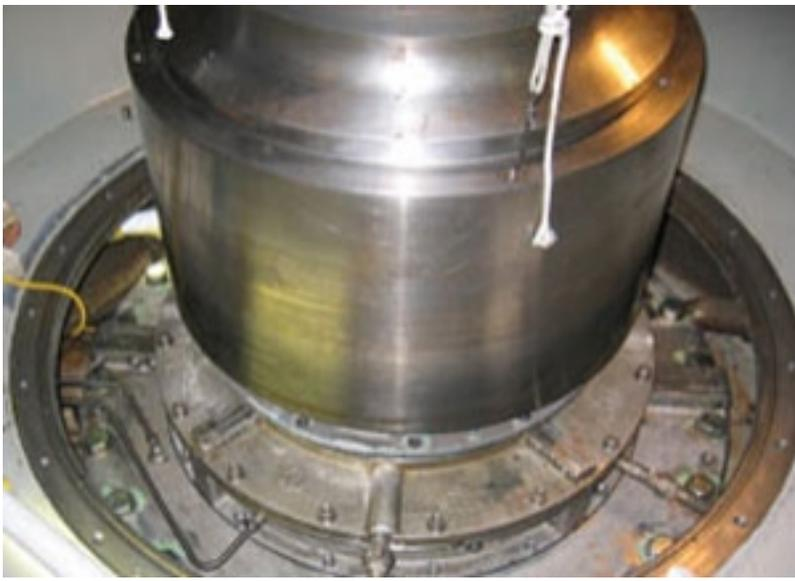
The new axial seal installed on this pump, at a facility in California, contains an innovative combination of face materials that can withstand severe applications. The old seal had to be replaced every three months; the new one has been in operation for three years.
